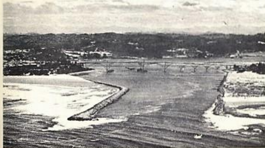
North jetty at Yaquina Bay is being extended 1,800 feet in a $5,376,000 project.
