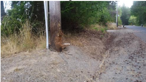
Gouged telephone pole
